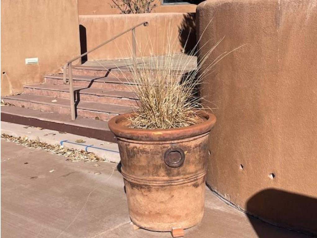
Picture #2: Planter Box on right-hand side of main entry steps. Note the 3 drain holes.
