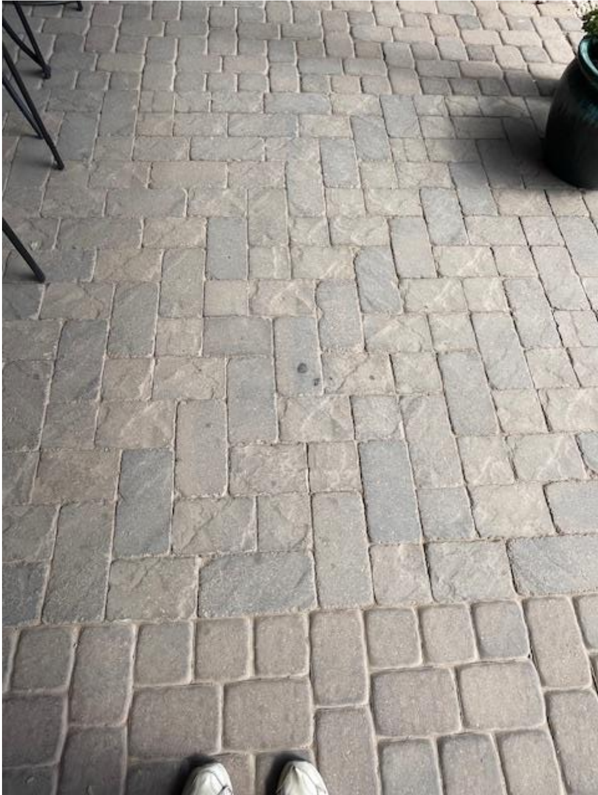
Example: Square-Rectangle Paver Layout. Pillow-topped surface.
