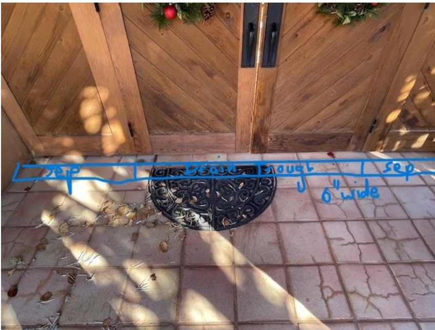
Picture #5: Location and dimensions of center drain trough and side separators.
